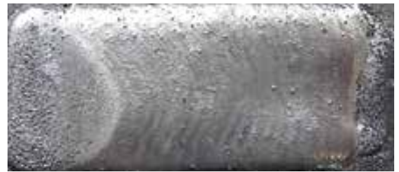
Typical welding joint
