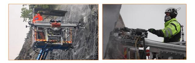
With drill rigs of Oprema Ravne operator works without physical loads present when drilling with hand tools. At the customer's request and by agreement, we can develop additional special sets or adjust the dimensions, number of drills... etc.
